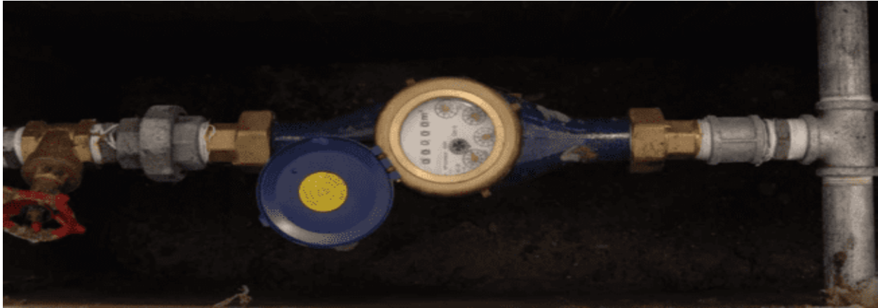
Figure 4: A newly installed Household meter in a House in Dar Es Salam
