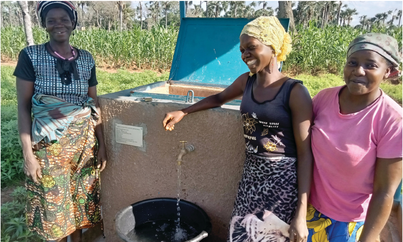
Community water supply at a public tap stand of Siniena village piped water network - Banfora commune. [Photo by Ismail KABORE / CRS]
