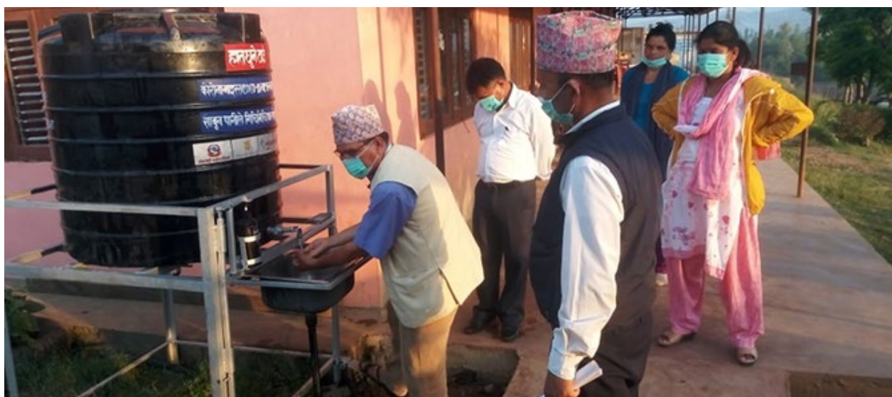
A locally manufactured, foot operated handwashing station is used outside a healthcare facility (Helvetas Nepal)
